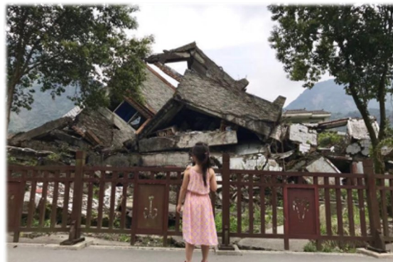
The debris of houses in Wenchuan after the earthquake
