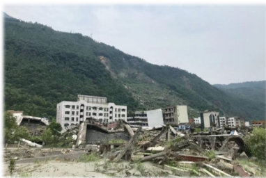
Houses in Wenchuan after the earthquake
